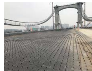
Location : Chengdu, China Project : Longwan Bridge Type : STC Bridge
