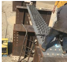
Location : Cairo, Egypt Project : Nile Bridge Type : Cross Rive Bridge
