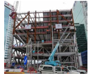
Location : Auckland, NZ Project : Commercial Bay Type : Shopping Center
