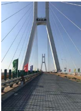
Location : Chengdu, China Project : Junshan BRidge Type : STC Bridge
